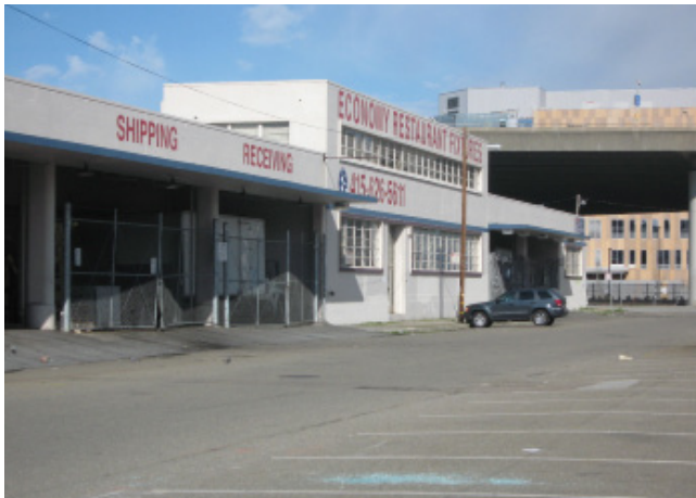
ABOVE: Many parcels of land are allocated to warehouses in the eastern portion of Showplace Square.
