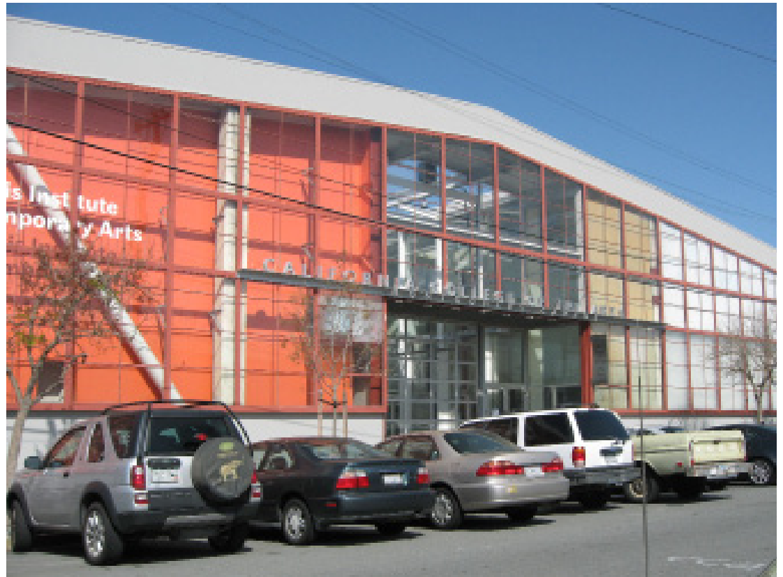
ABOVE: The California College of the Arts Campus (CCA) serves students in the architecture and design fields. The building holds several design studios and a lecture hall. The CCA on 8th Street is home to the Wattis Gallery, and A^2 Cafe.
