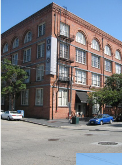
LEFT and BELOW: Galleries and showcase warehouses are scattered throughout the area.
