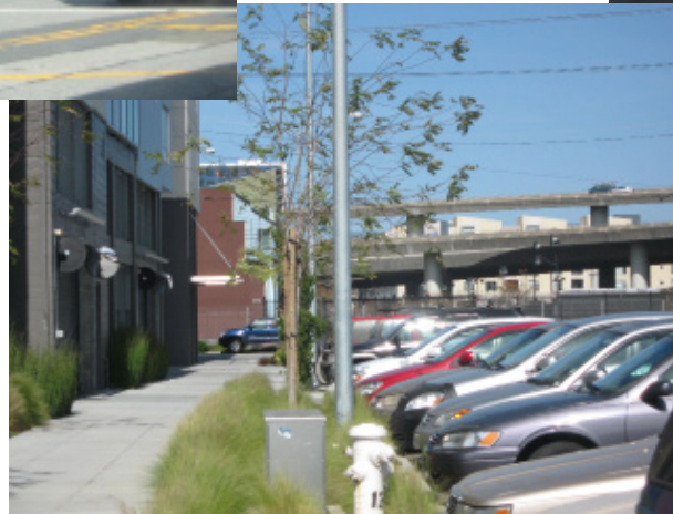
RIGHT: Bioswales are implemented in the parking lot of the new mixed use development.
