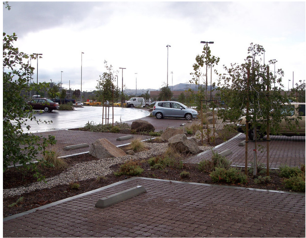
FIG 3.12 The parking lot at the El Rio de Los Angeles State Park has many stormwater facilities.
