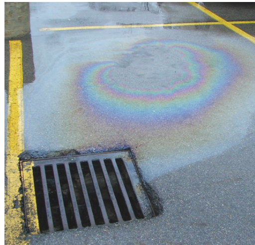
FIG 2.4 Oil spills and other sediment from cars sits on the surface of impervious parking lots.
