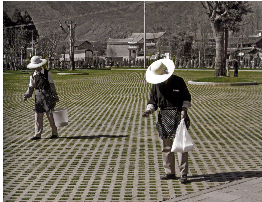
FIG 3.12 The parking lot at the El Rio de Los Angeles State Park has many stormwater facilities.
