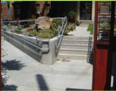
Top to bottom: Figure 1.35—View of Comfort Garden towards Potrero Avenue Figure 1.36—Stairs and ADA ramp at southwest corner
