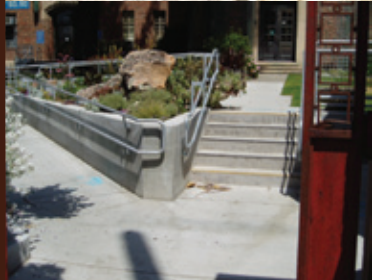
Top to bottom: Figure 2.9—Colorful, dense plantings at UCDMC Urban Wildlife Preserve; Figure 2.10—Handrails available for patients having trouble walking; Figure 2.11—Effective use of textures at UCDMC Wildlife Preserve; Figure 2.12—Stairs and ADA ramp at Comfort Garden
