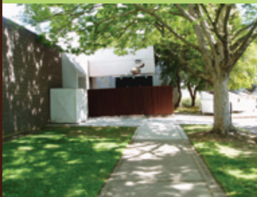
Top to bottom: Figure 1.70—Southern Side of building Figure 1.71—Northern Side of building Figure 1.72—Western Side of building
