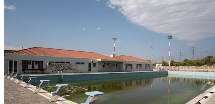
Figure 1.2 Abandoned swimming pool
