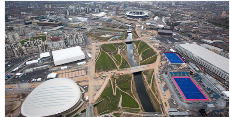
Figure 1.10 An aerial view of the Olympic Park
