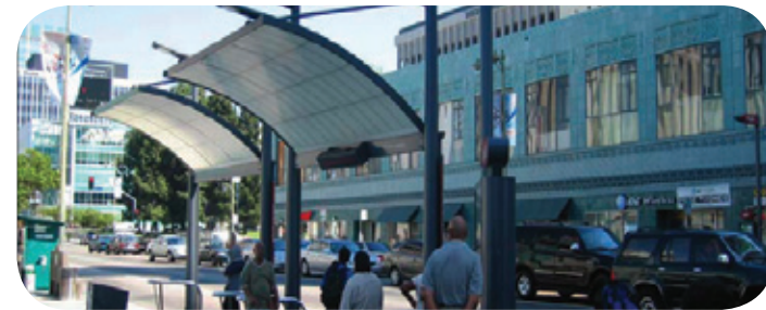
Figure 2.26: Image of an Orange Line station. Image of what I think is a poor station shelter.
