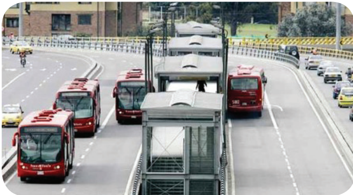
Figure 1.24B: Passing Lanes at Stations
