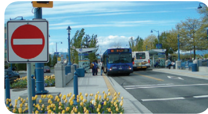
Figure 1.23B: Extended Platform Without Assigned Berths
