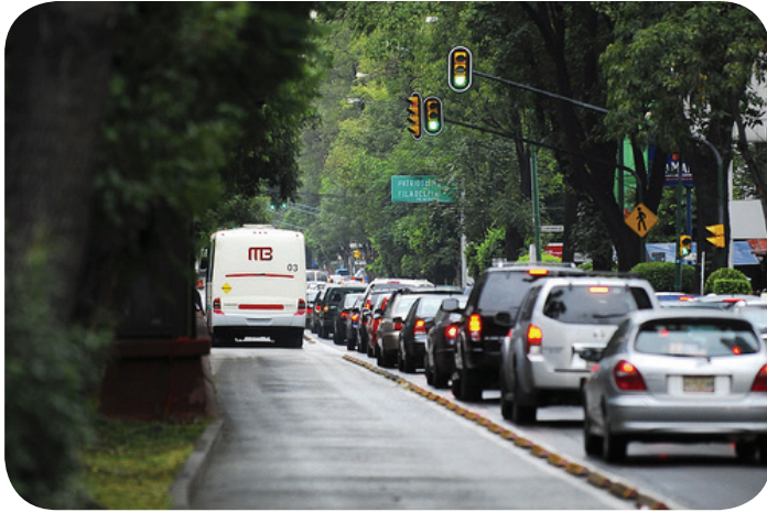
Figure 1.16: Raised Lane Delineators in Mexico City
