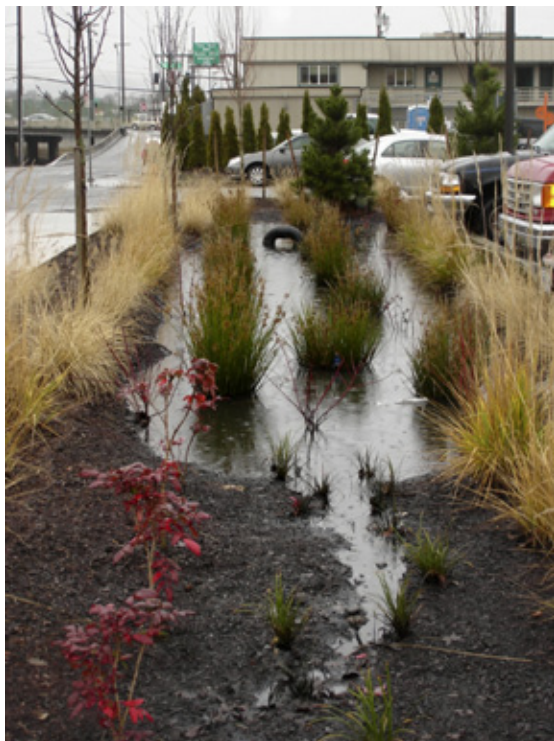
3.1 - Runoff collecting in a swale, Portland, Oregon (oregonlive.com)
