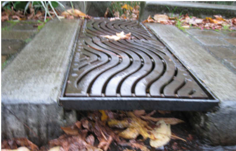
6.12 - SW 12th Ave. inlet
