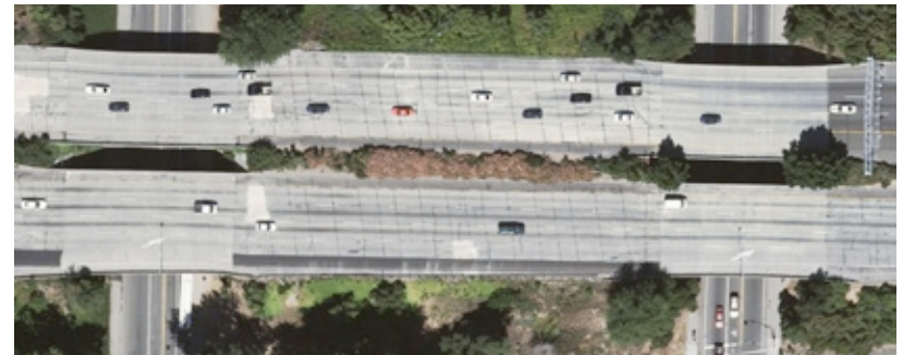
5.1 - Capitol City Freeway, Sacramento, CA (Google Earth)
