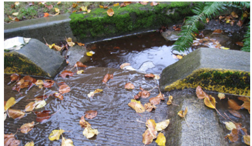
6.7 - Stormwater planter curb-cut
