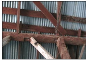
fig. 9 North Barn Rafters
