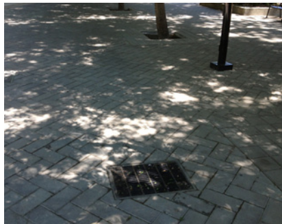
STORM DRAINS (North)
