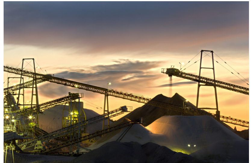
Fig. 2.7 - The industrial infrastructure for mining
