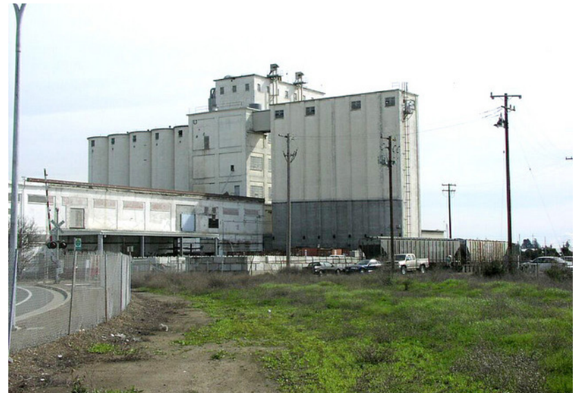
Fig 3.4 - Industrial area adjacent to Union Point Park
