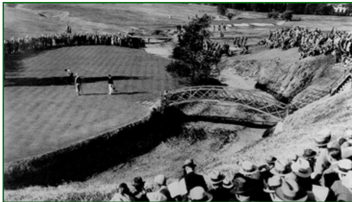
Figure 14. 18th green at Wilshire C.C., Los Angeles. To protect the green, this arroyo now is lined with a rectilinear concrete liner.
