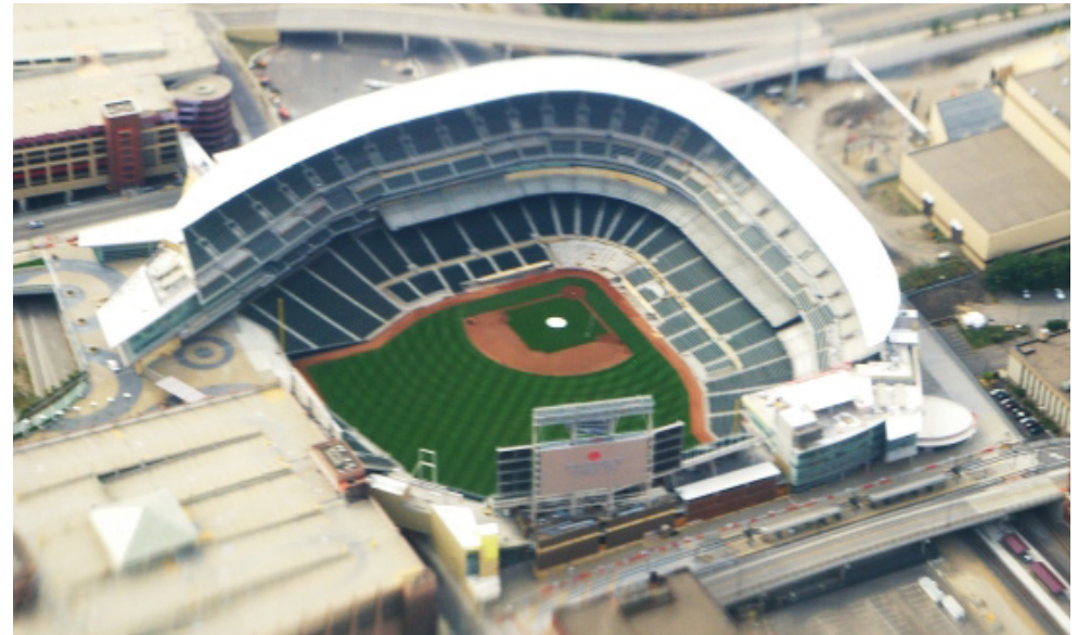
FIGURE 2.32: Aerial of Target Field and Its Rain Collecting Roof Top
