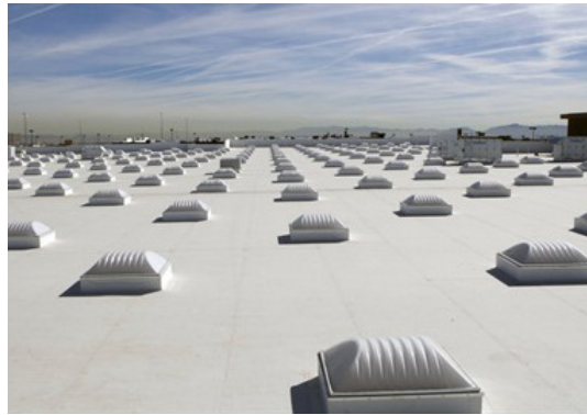
FIGURE 2.18: White Roof On Top of Walmart
