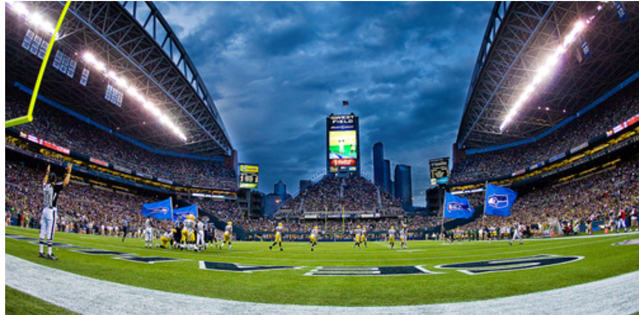
FIGURE 2.35: Seahawks Stadium At Night
