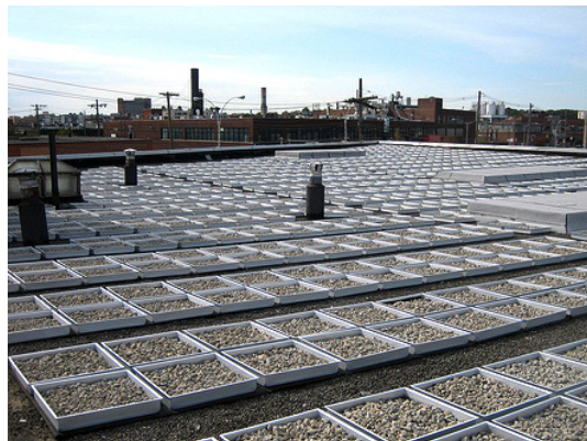
FIGURE 2.17: Blue Roof in NYC
