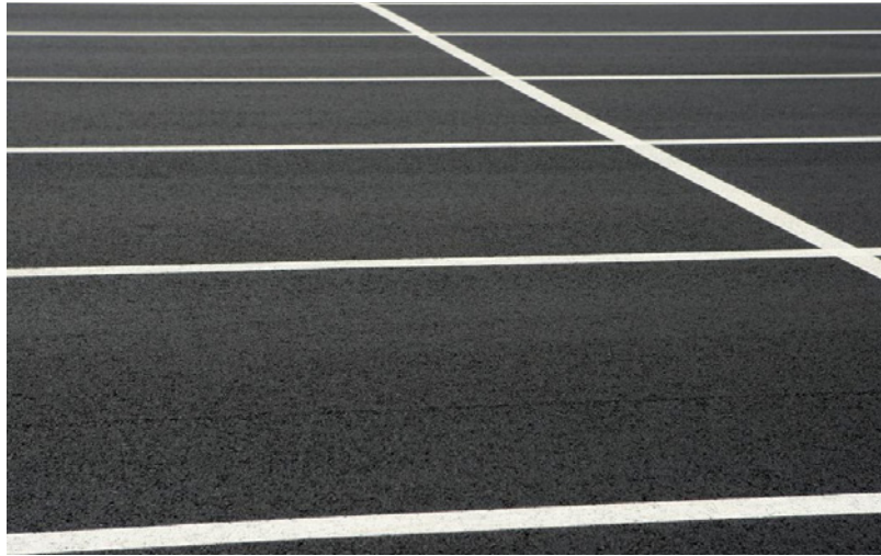
FIGURE 2.10: Typical Asphalt Parking
