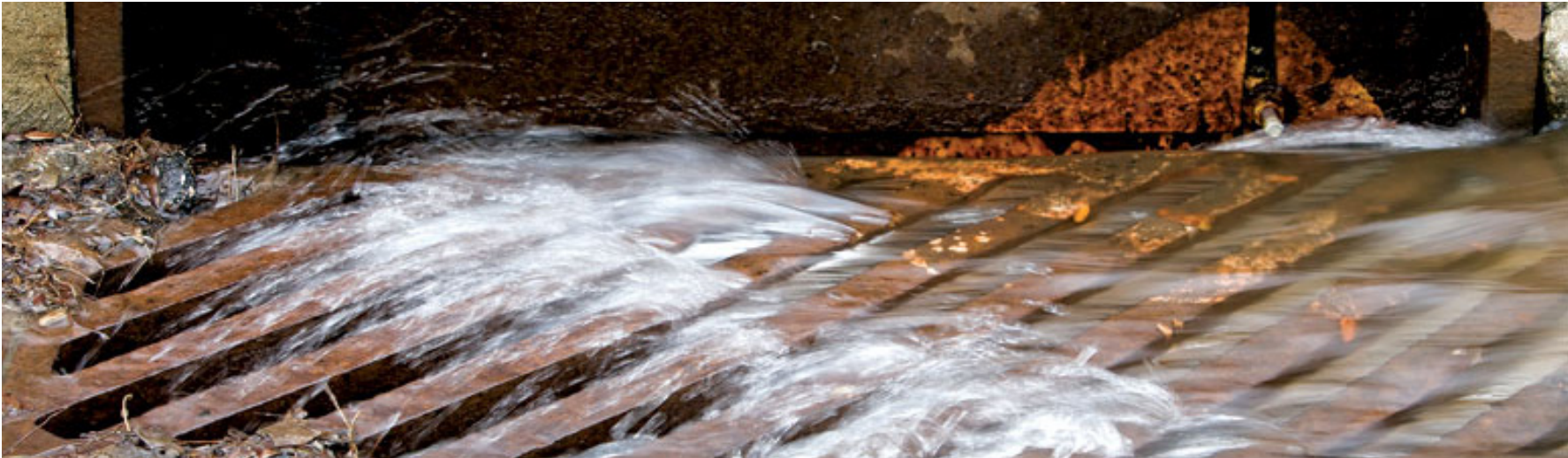
FIGURE 2.28: Storm Water Runoff Going Straight to a Drain Inlet
