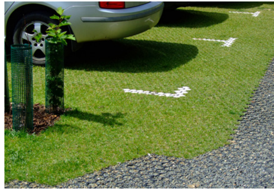
FIGURE 2.13: Grass Containing Reinforced Grid Systems
