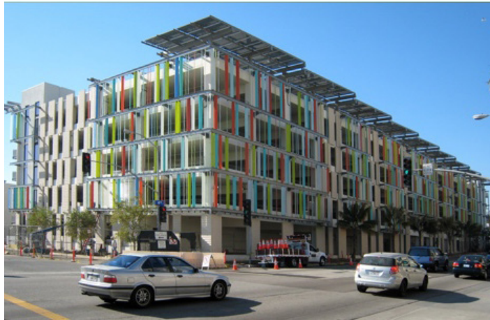
FIGURE 2.47: Street View Of the LEED Garage
