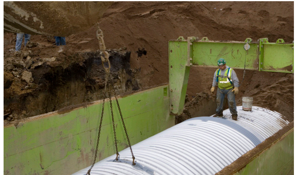
FIGURE 2.33: Installation of the Underground Cistern
