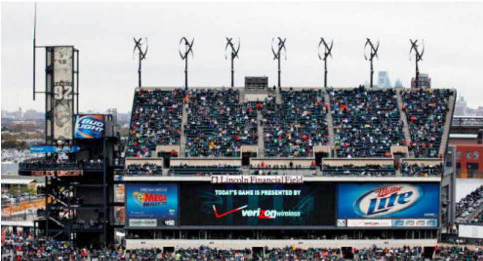
FIGURE 2.43: Wind Turbines Within the Facility
