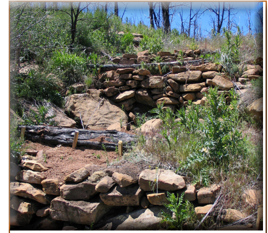
Native American check dams kept silt and water behind the wall for farming into the dry season with the moisture stored in the soil
