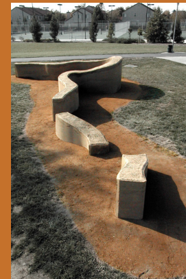
Troy Corliss' rammed earth design recalls the meander of the North Fork of Putah Creek. The material he chose would be appropriate for earthworks. citation a.
