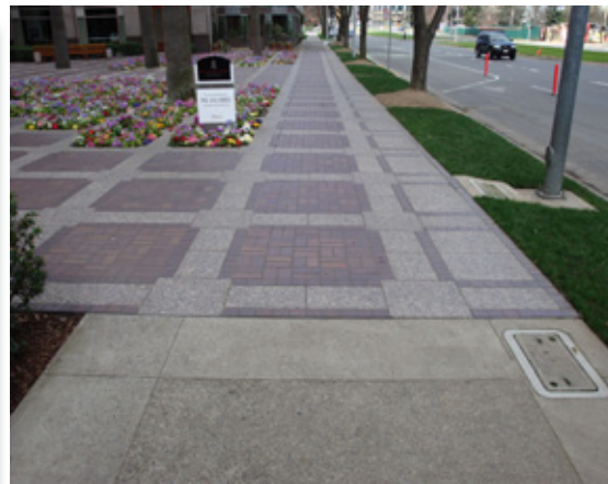
Wells Fargo Building Entry Plaza
