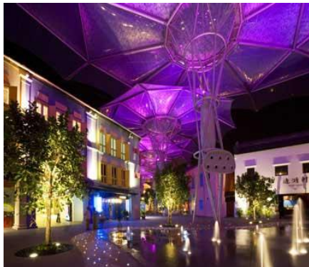
Fig. 33 – Canopies, Fountain, and Lighting
