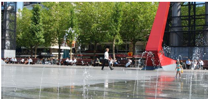
Fig. 36 – Water Feature and Cooling Towers
