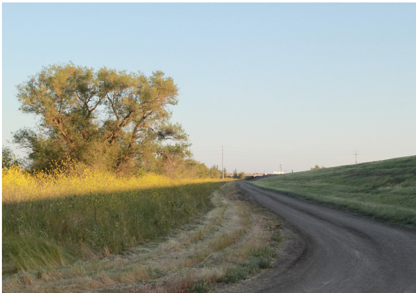
Figure 35.2 - Fine line between riparian areas and levee vegetation. Levees are completely disturbed and often harbor invasive weed species. There is a great opportunity to use these disrupted landscapes for habitat restoration
