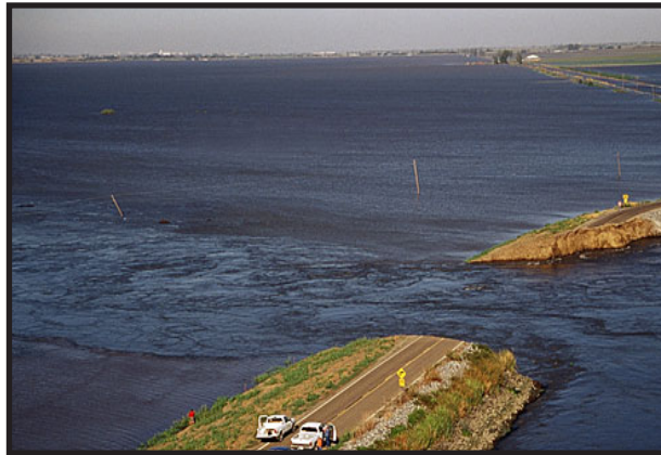
Figure 12. - Levee breach at Jones Tract in 2004 that occurred on a normal sunny day (DWR, 2009).
