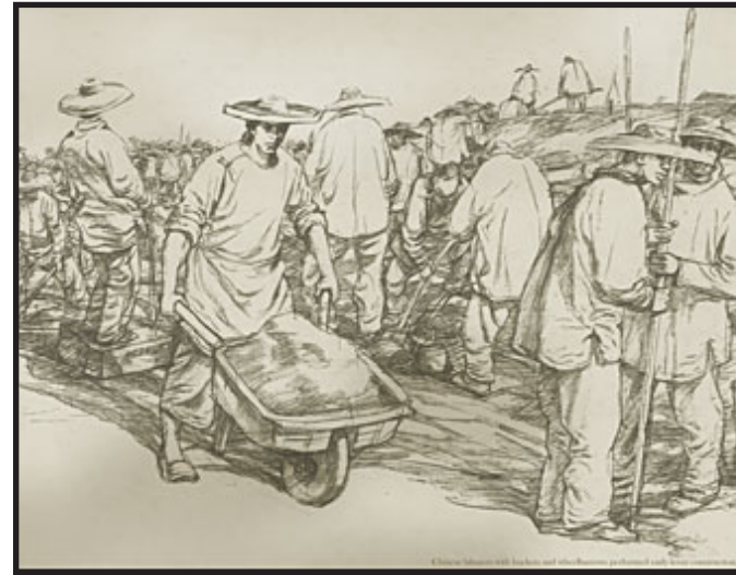
Figure 7. - Chinese laborers constructing levees with wheelbarrow and shovels. (Department of Water Resources, 2012)
