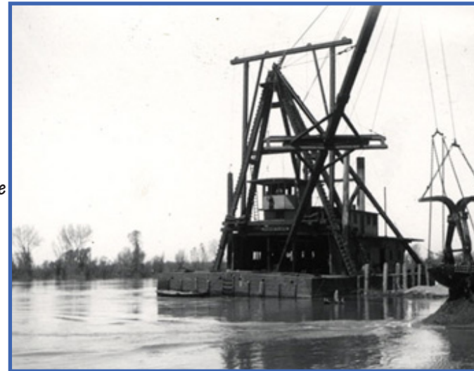
Figure 8. - A sidedraft - clamshell dredger removing sediments from the river to construct a levee (Department of Water Resources 2012).
