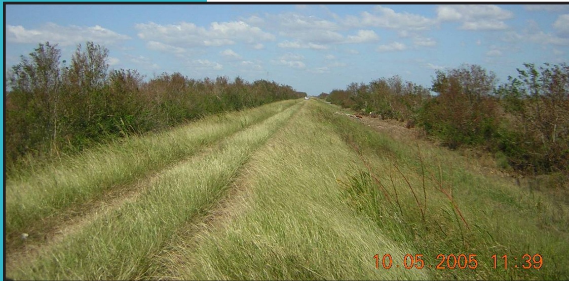
Figure 27. - A stretch of a vegetated levee in New Orleans that was virtually unchanged by the events of Hurricane Katrina (Source: Berkeley Independent Investigation Team, 2006)
