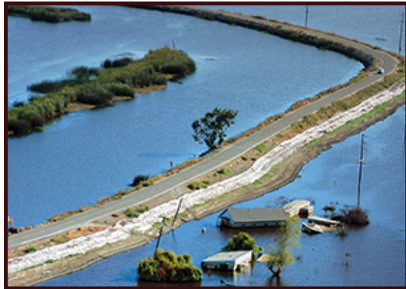
Figure 11. - Levee Failure at Jones Tract showing property destruction (University of California Davis, 2007)
