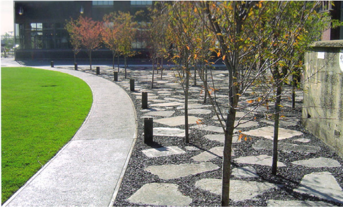
Figure AB. Example of concrete reuse. Courtesy Living Systems.
