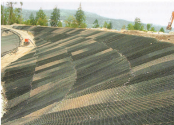
Figure W. Envirogrid used for structural approach. Courtesy Living Systems.
