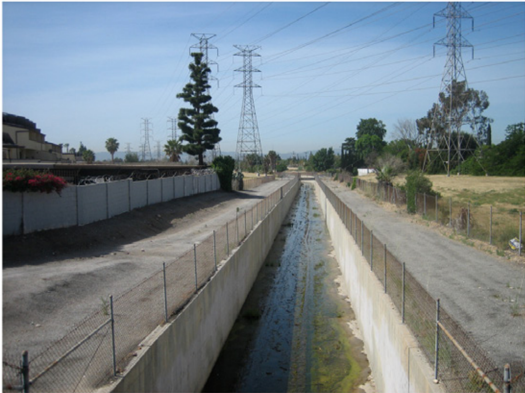
ALISO CANYON - BEFORE REHABILITATION
