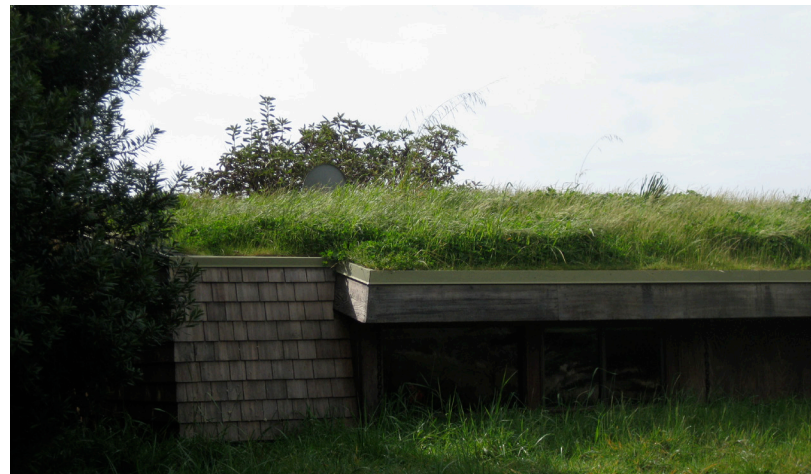
Fig. 41: Mounding on Green Roof Levy, S., 2012
