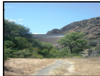
5. View of Monticello Dam from the western portion of the site.
