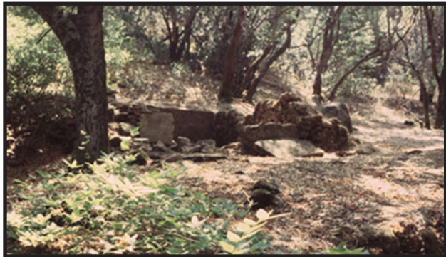
Fig. 2.3 Cold storage foundation, Vlahos Homestead
