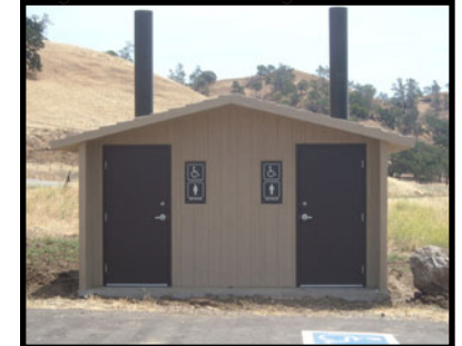
Fig. Fishing access vault toilets
