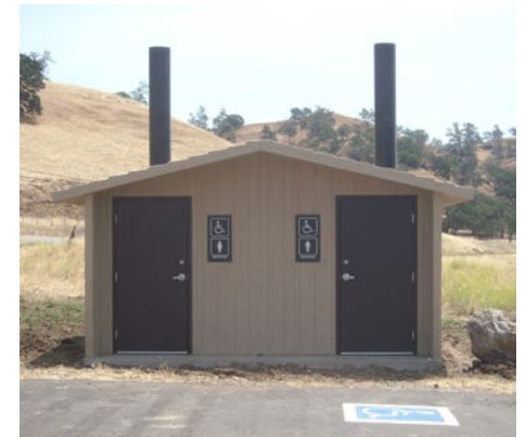
Vault Toilets are located in next to the main parking area.
