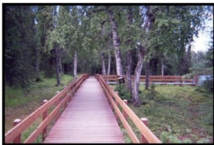
Ramp to the pier
