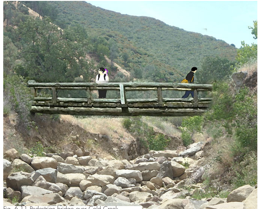
Fig. 6.11 Pedestrian bridge over Cold Creek
