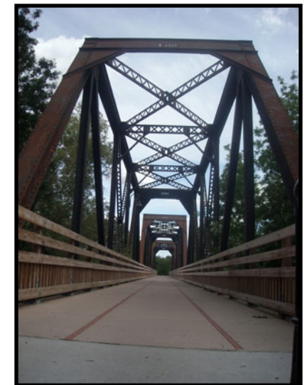
Fig.5.12 The Railroad Bridge
