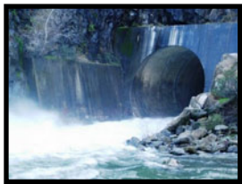
Fig. 1.20 Glory Hole spillway exit
