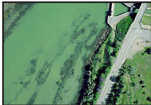
Fig. 1.21 Putah Diversion Dam
