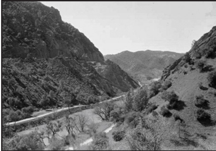
Fig. 1.16 Devils Gate before Monticello Dam
