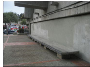
Abandoned seating area
