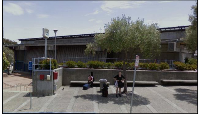
Fig. 26 Upper plaza seating area
