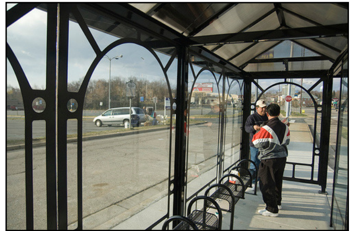
Fig. 36 New bus and street car shelters in Toronto
