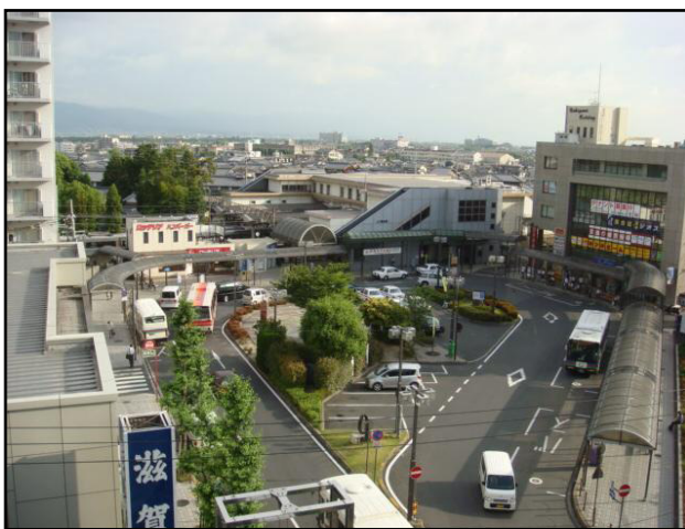
Fig.1 Seta Train Station
