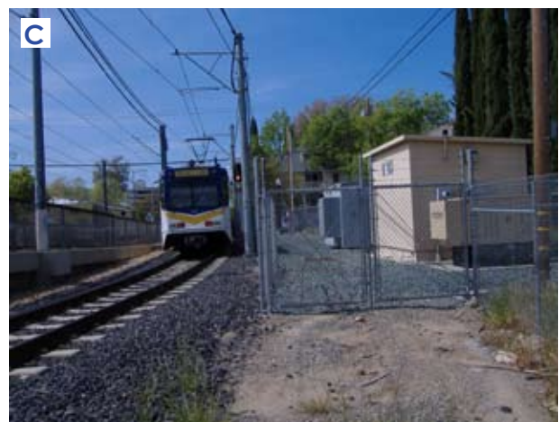
View west along the light rail tracks .
