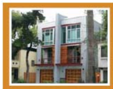
7. Q Street Lofts
