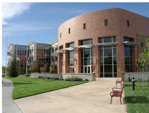
Figure 2.5 West Sacramento City Hall.
