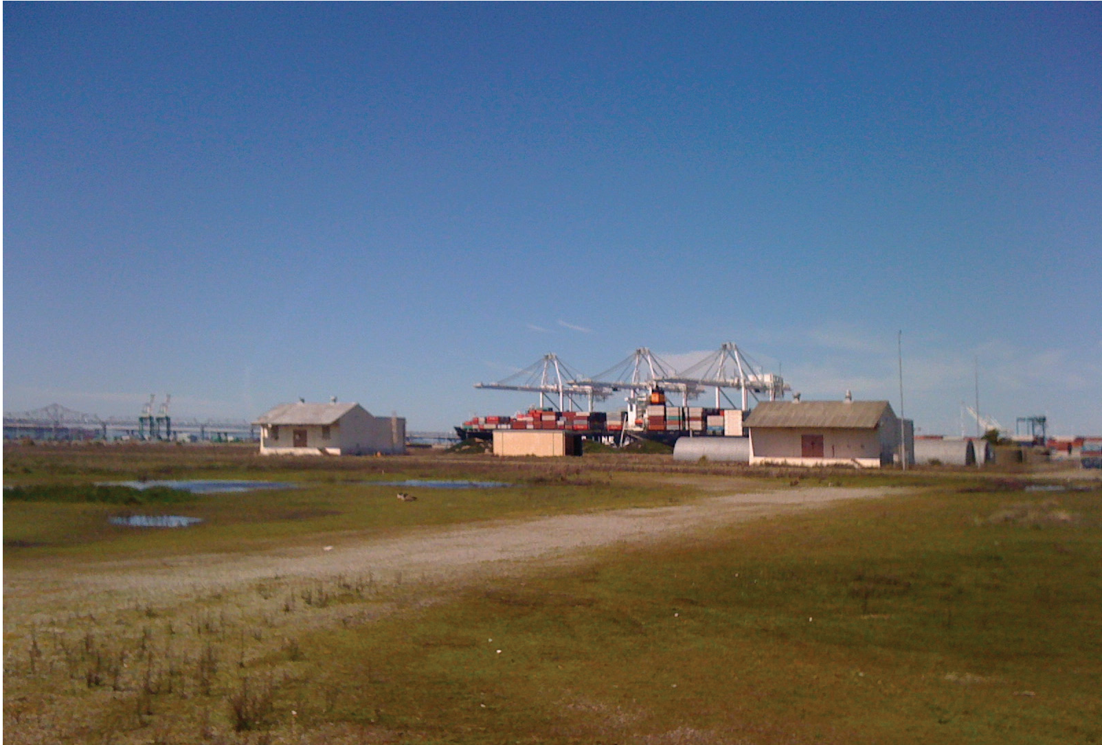
Fig 35 View towards north west end. (Source: Thompson)
