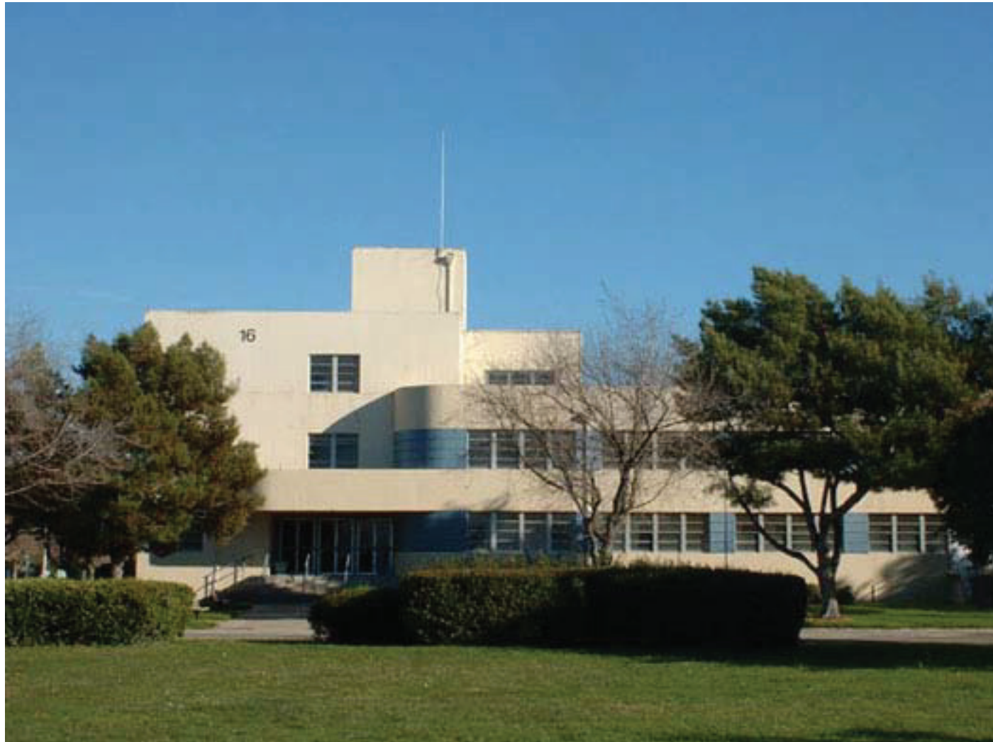
Fig 25 Administrative core. (Source: Historic Survey)
