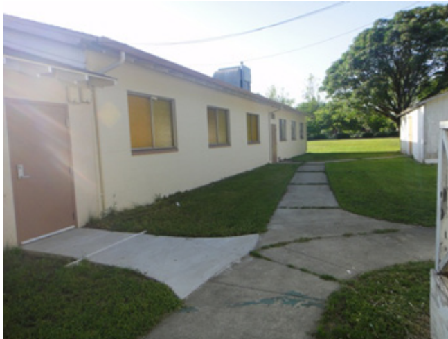
Above: Site photo of existing pathway.
