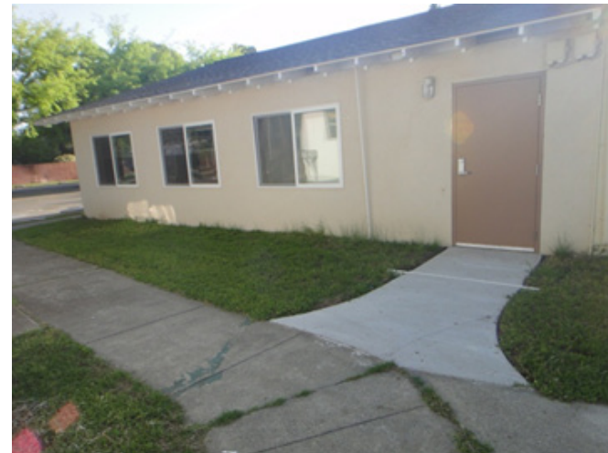
Above: Site photo of existing pathway.
