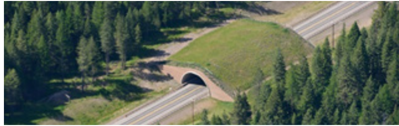
Figure 5-2 Wildlife overpass crossing U.S. 93 (Montana Department of Transportation et al., 2000)
