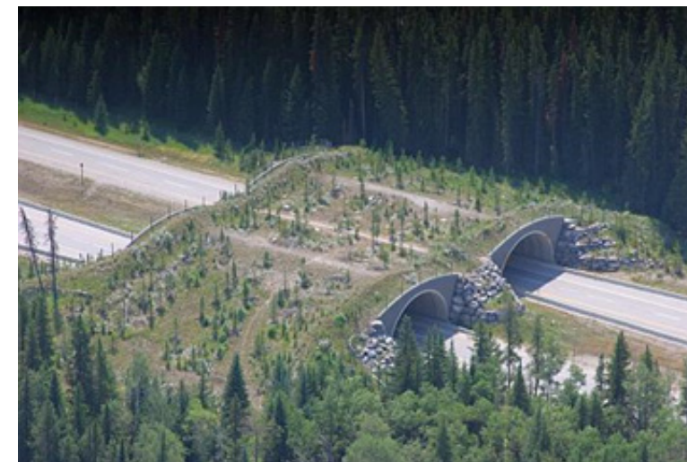
Figure 5-5 Wildlife overpass at Banff National Park (Segal, 2018)
