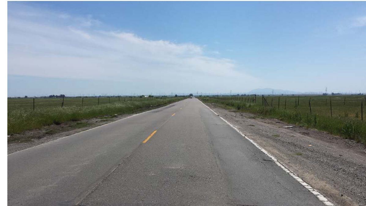
Figure 6-8 Highway 113, facing South (Gee, 2018)
