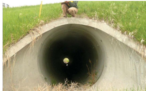
Figure 4-9 Small- to medium-sized underpass (Federal Highway Administration, 2011)
