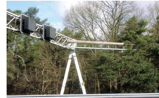
Figure 4-4 Canopy crossing (Federal Highway Administration, 2011)
