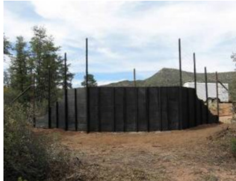
Figure 4-14 Wildlife escape ramp, rear view (Arizona Department of Transportation)
