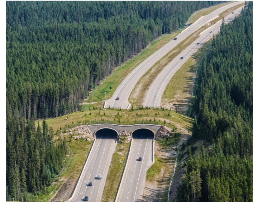
Figure 5-1 One of six wildlife overpasses at Banff National Park, Canada (Conservation 2020)
