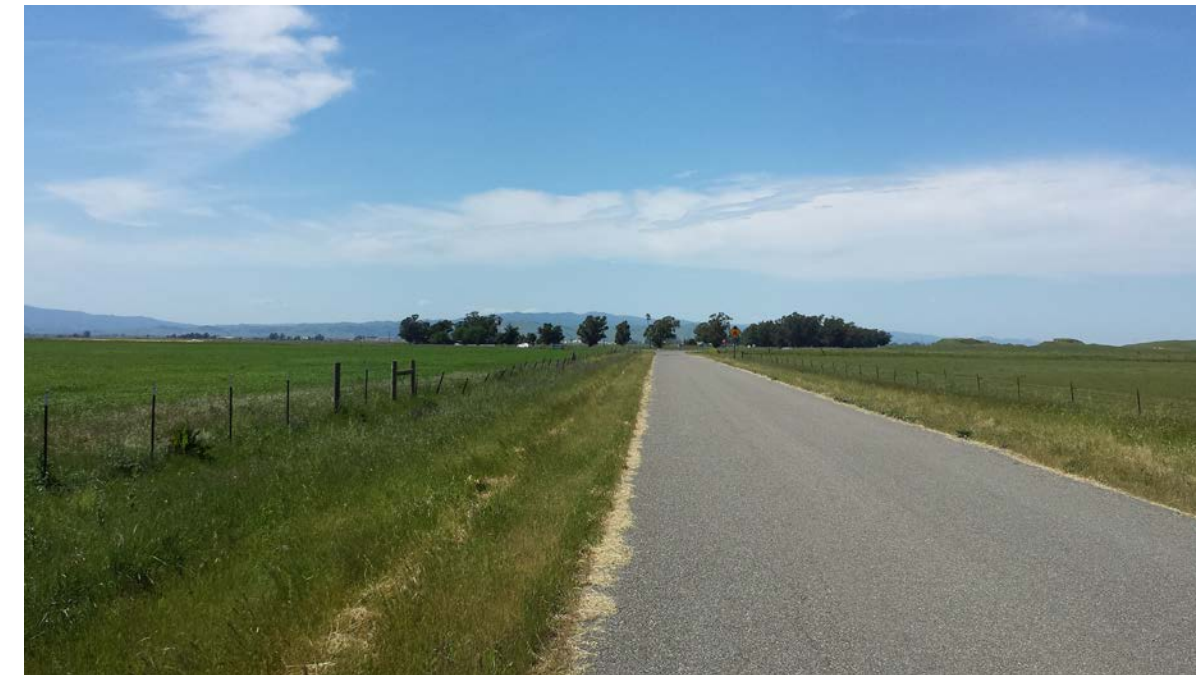
Figure 6-6 Highway 12, facing West (Gee, 2018)
