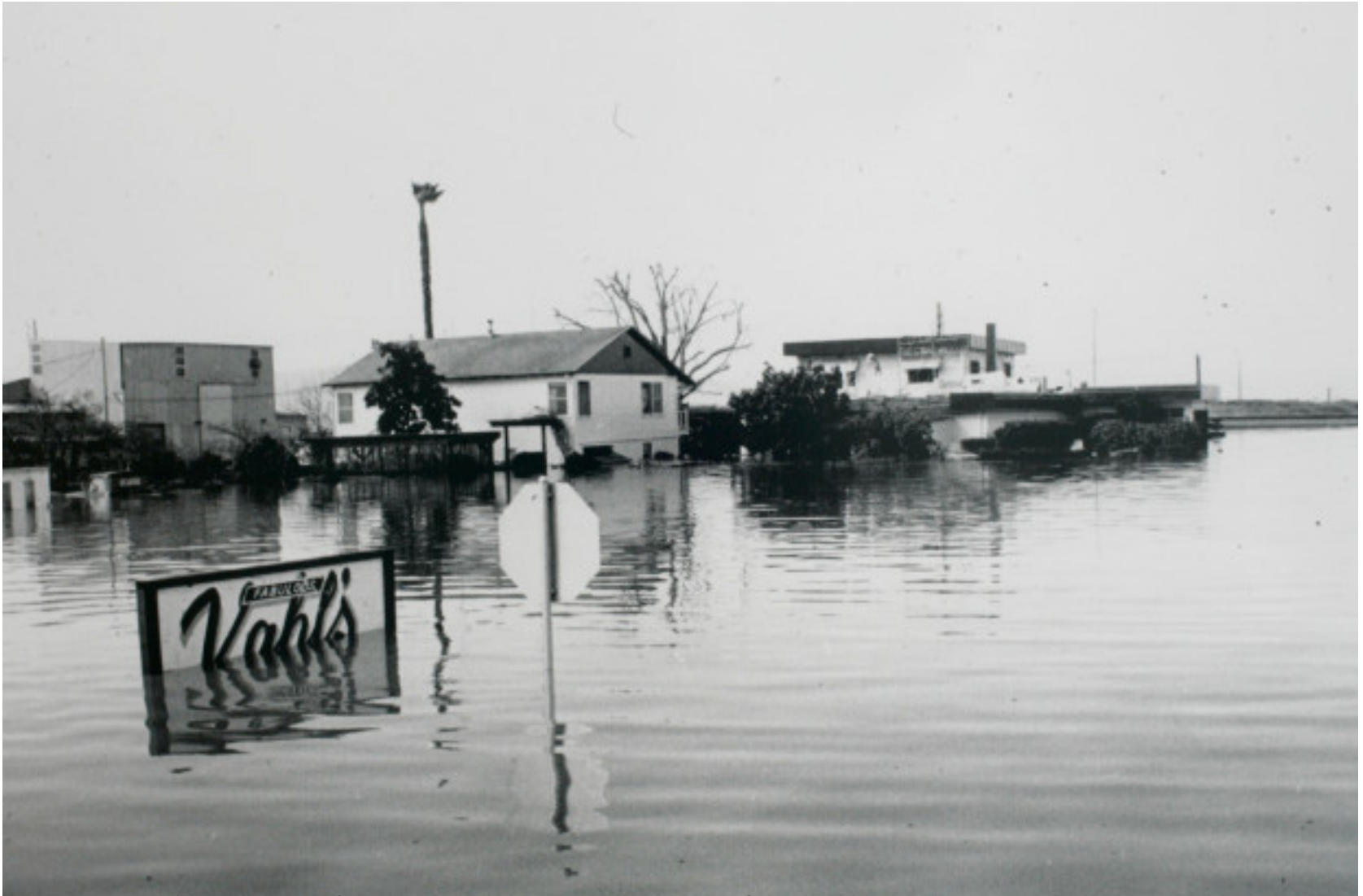
Figure 11. Alviso's most severe floating due to storm surge and non-functional levee design 1983
