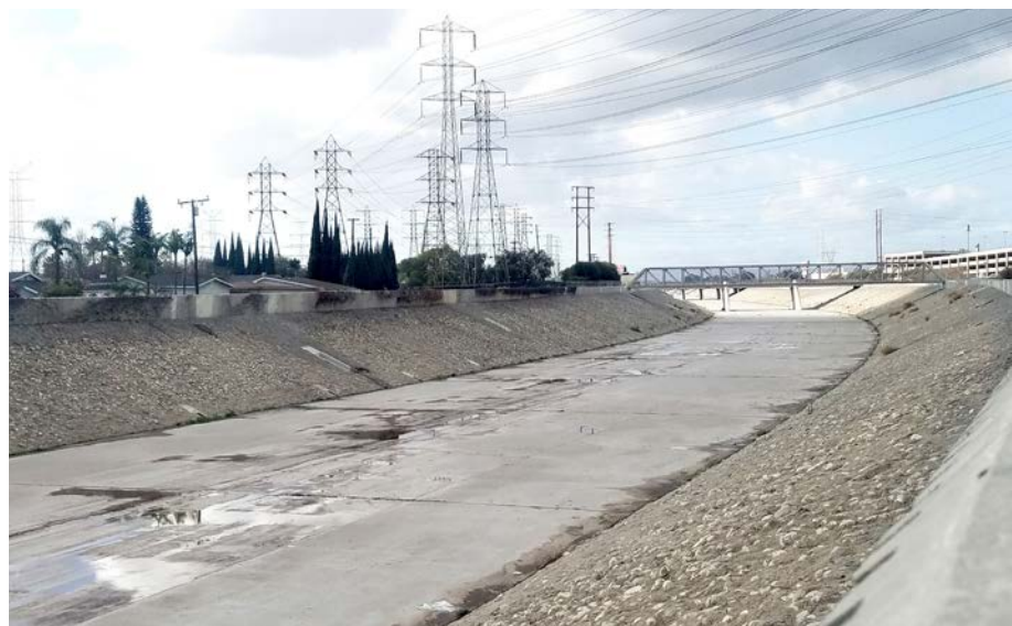
Figure 22 : Rio Hondo Canal is prominently encased in concrete. Photography by: Karen Lomas-Gutierrez
