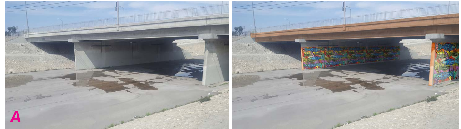
Figure 83 : Before and After view of vehicular bridge after adding some color to the gray walls
