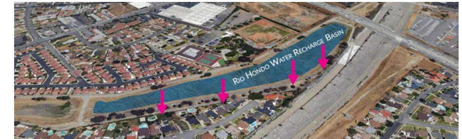
Figure 64 : Rio Hondo Spreading Grounds functions as water recharge basin. Image Source: Google Earth
