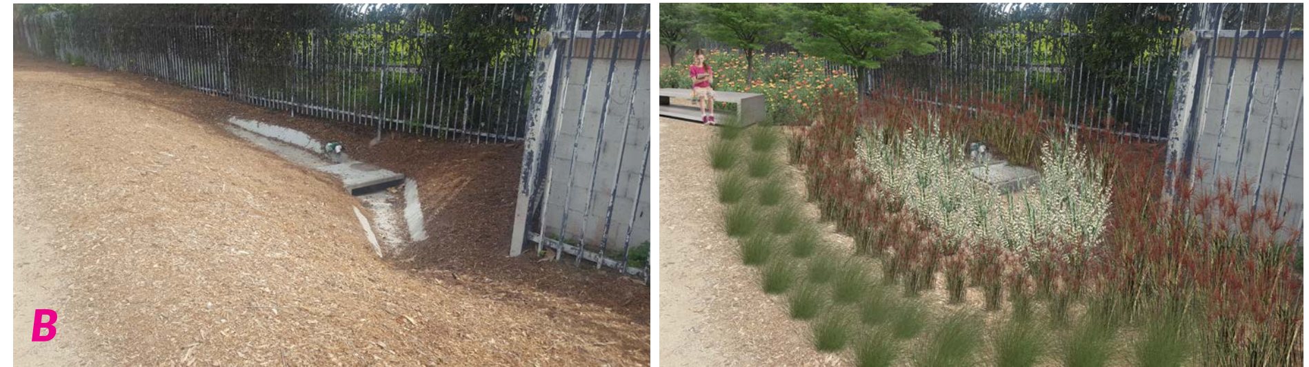
Figure 84 : Before and After view stormwater drain after transforming it to a rain garden
